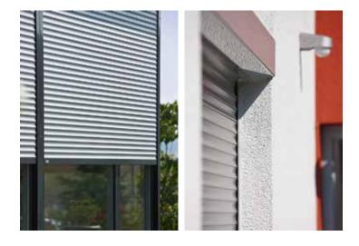
**Multi-talented front-mounted roller shutters:** the Varimaxx system is a subtle universal genius with inner and outer values. The design with the "added angle" always creates a soft uncluttered finish to your window. It is square without appearing awkward or angular. The straight lines of the roller shutter box become one with the style of every building.
